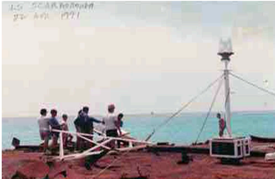
Figure 10. The automated light station installed by the Philippines on Scarborough Shoal, circa 1991, to replace a lighthouse built earlier. 75
